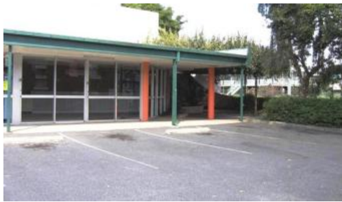
SHOP 1, 12 South Station Rd, Booval
