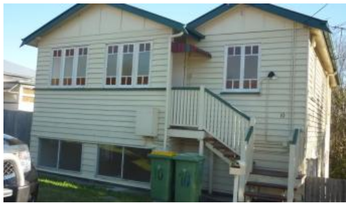
10 Gulland Street, North Ipswich
