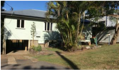
Unit 1, 4 Harold Street, Bundamba
