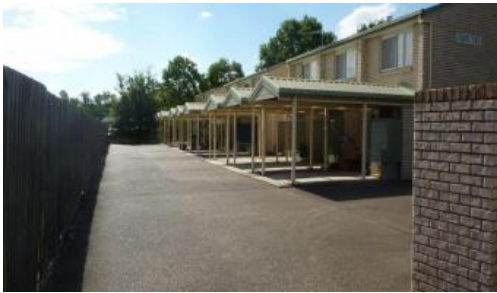
Unit 8, 16 Lindsay Street, Bundamba
