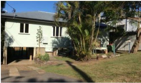
Unit 1, 4 Harold Street, Bundamba
